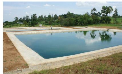
OXIDATION POND FOUR(4) IN NUMBER
